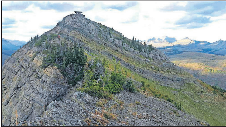
WHILE NOT currently staffed, the fire lookout on Heaven's Peak in Glacier National Park was assessed for maintenance needs this summer. (photo provided)
