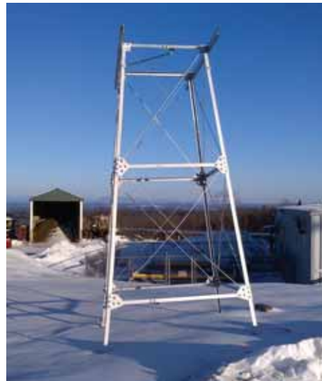
Squaw Mountain steelwork stripped and painted (Sam Bradeen photo)
